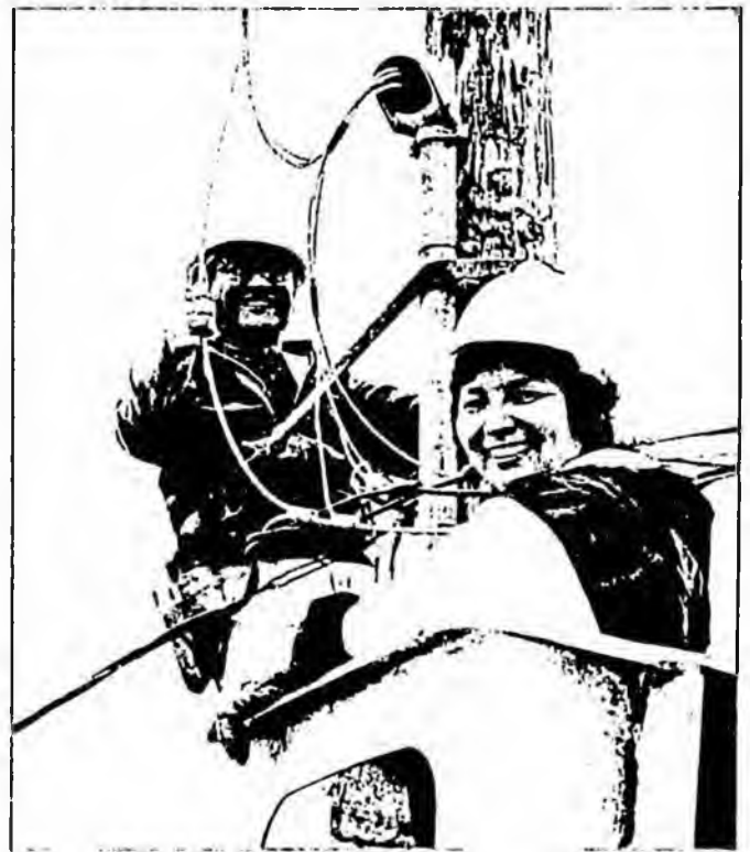
Two utility workers inspecting a power pole. Photo courtesy of WEA.
