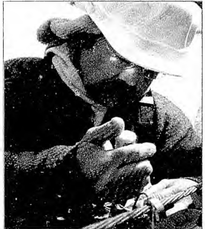
An Arctic Slope Telephone Association Cooperative, Inc. (ASTAC) telephone technician splices wires. Photo is courtesy of ASTAC.
