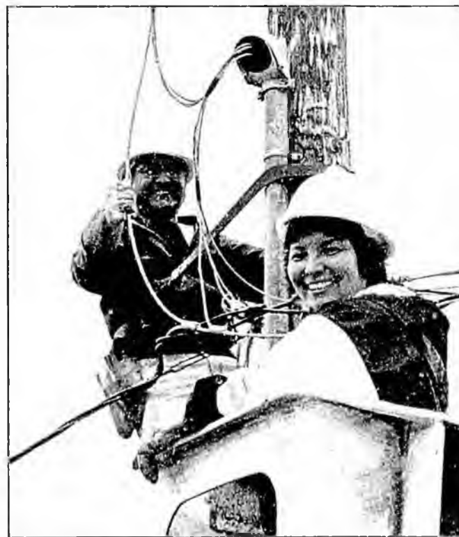
Alaska Power & Telephone Company (AP&T) Metlakatla crew (Richard Booth and Kathy Brendible) are shown working on a power pole. Photo is courtesy of AP&T.
