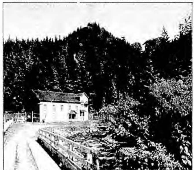
Taken out of service in 1998, this is one of two power houses built to generate power that used water from the Salmon Creek Dam. Photo is courtesy of Alaska Electric Light & Power Company.
