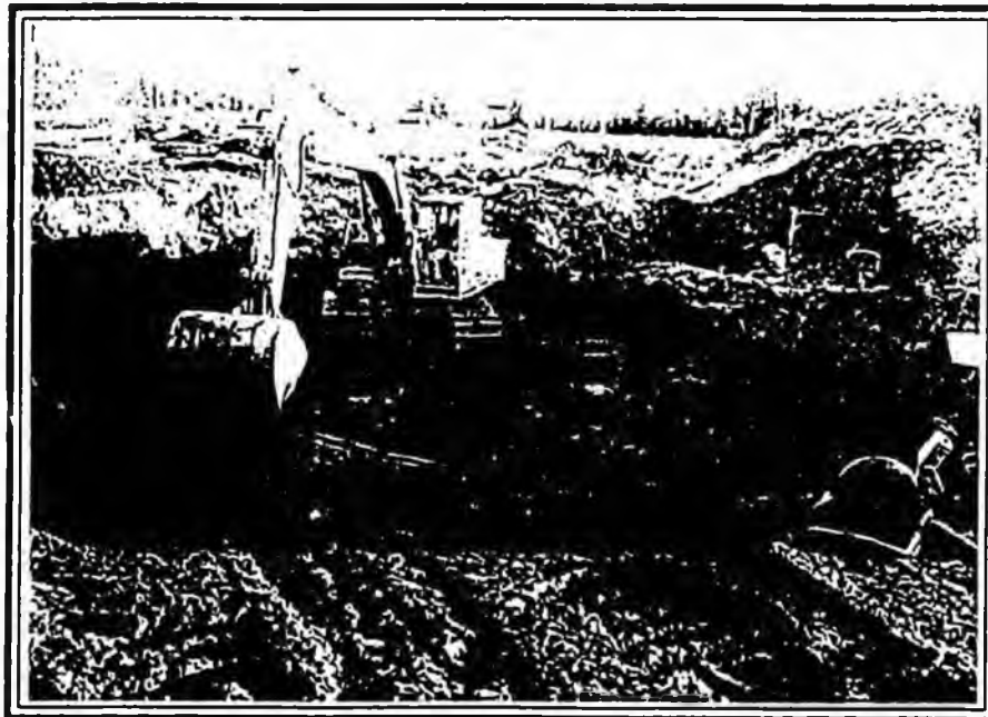
Sterling facility undergoing cleanup activities.
