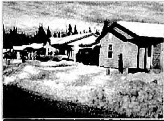
Mooring Estates, Soldotna FY1996
