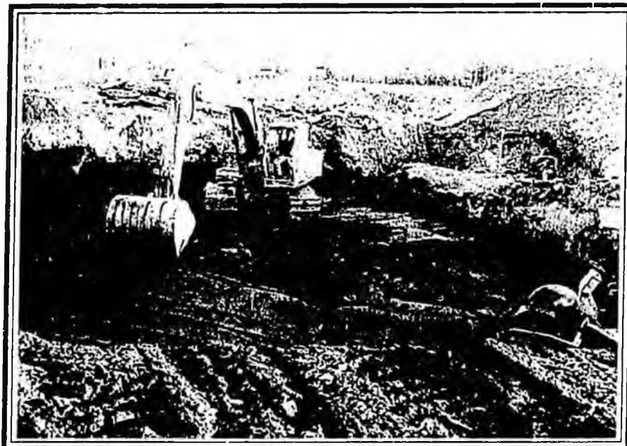
Sterling facility undergoing cleanup activities.
