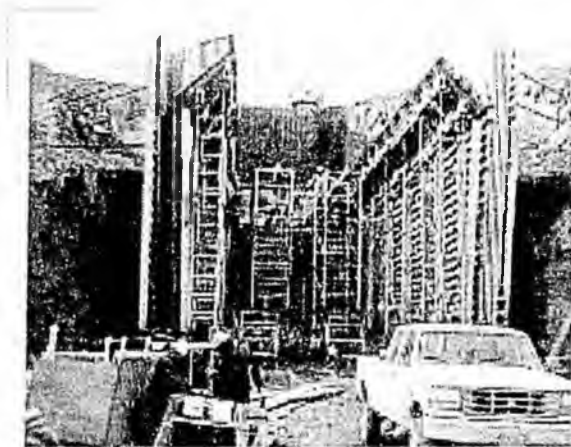
Flame Trench for the Launch Pad
