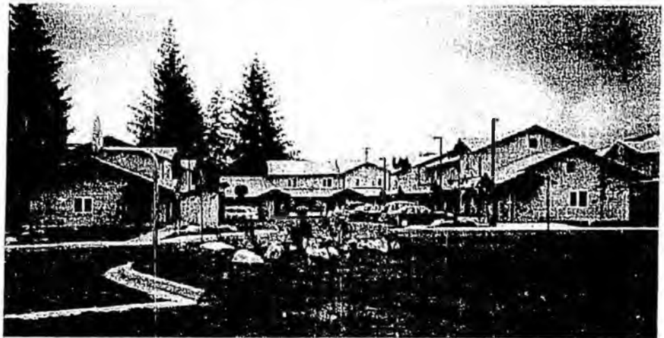
AHFC's Public Housing Division received a NAHRO design award for Riverbend, a 45 unit public housing complex built in Juneau in 1998.
