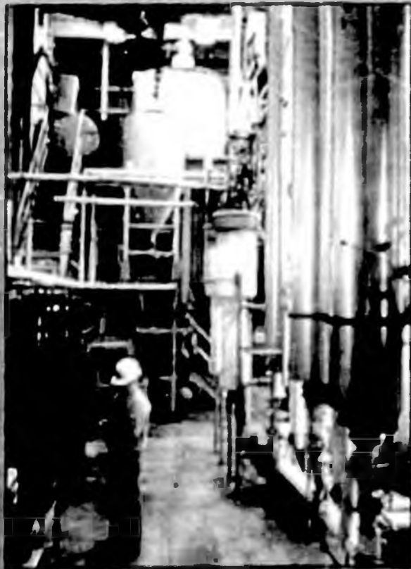
BERC HVD Plant
