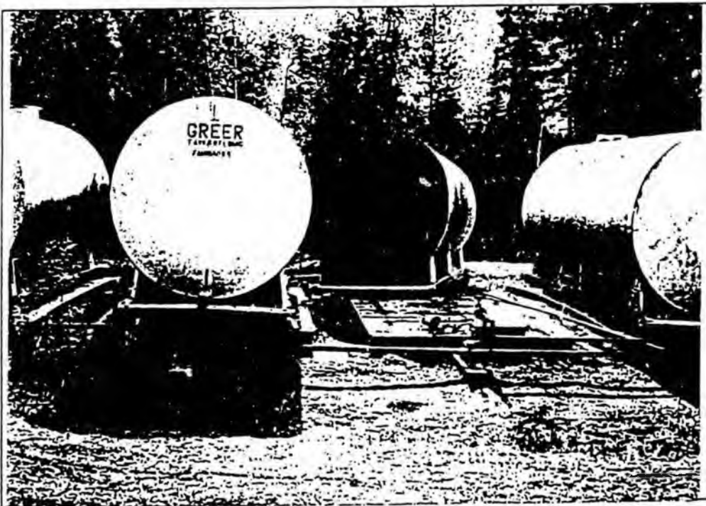
Photograph A.8 Improper piping system and poor operational procedures resulted in explosion of tank.
