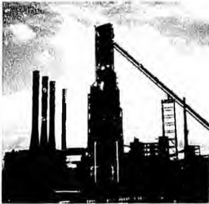
Essar Steel plant in Hazira, India. (top photo)
