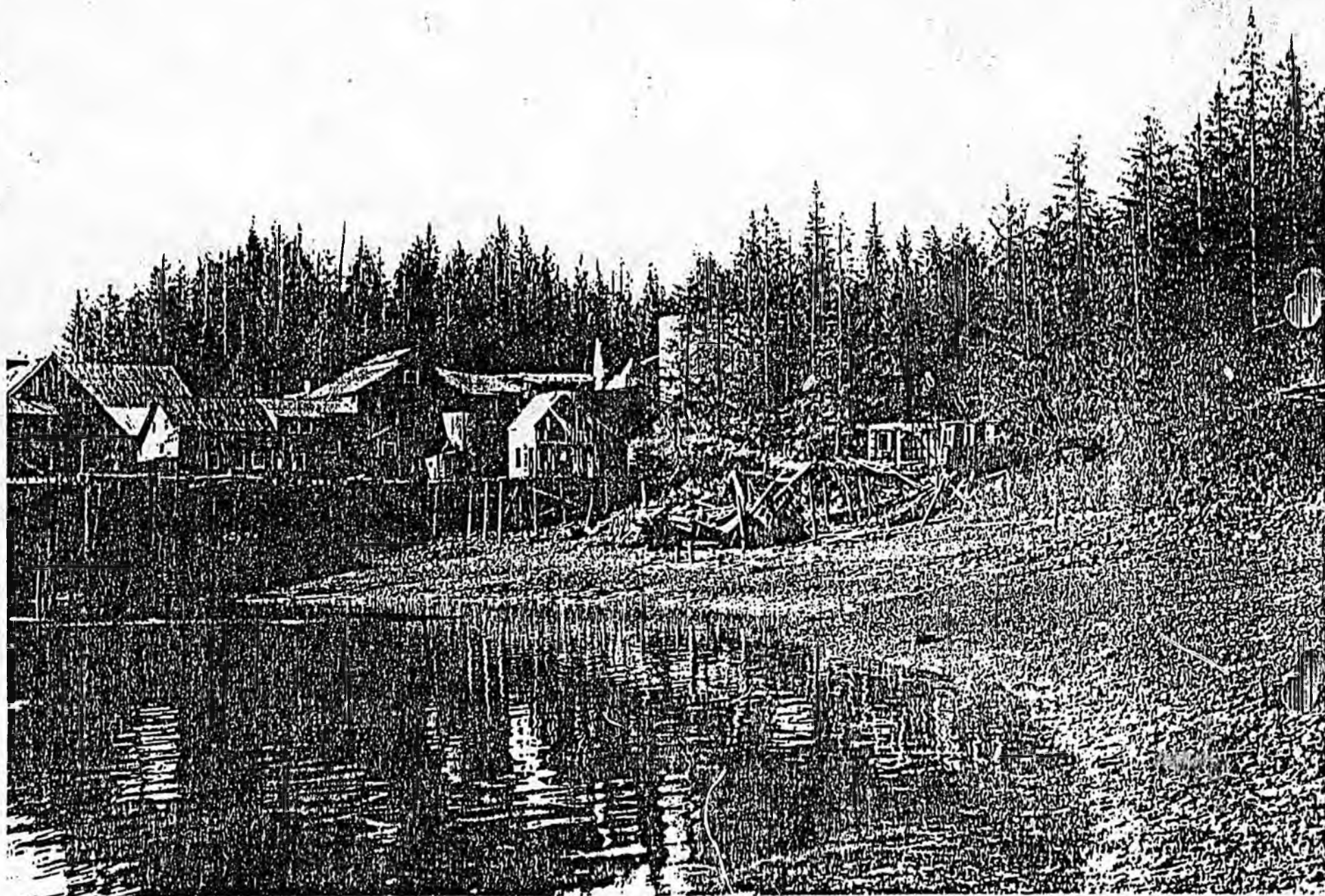
PHOTO #3. Cannery damaged during and abandoned after 1964 earthquake (uplift in area 8 to 9 feet).
