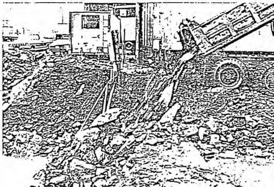
Photo No. 11: View as per Photo No. 10 above. Emergency rock fill being placed to prevent further spalling of bank.
