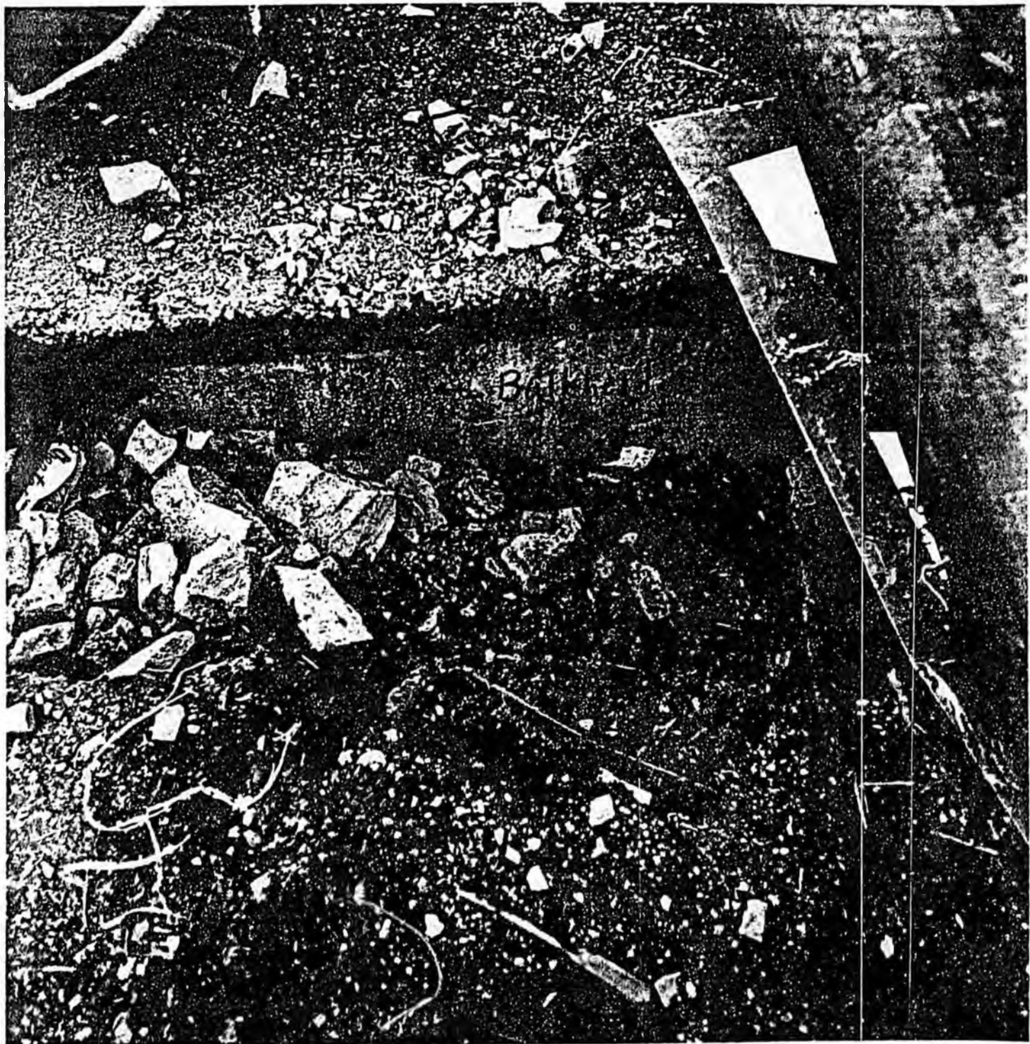
Kodiak, Alaska PIER 3 Near East end of wharf on or about 1-28-80
