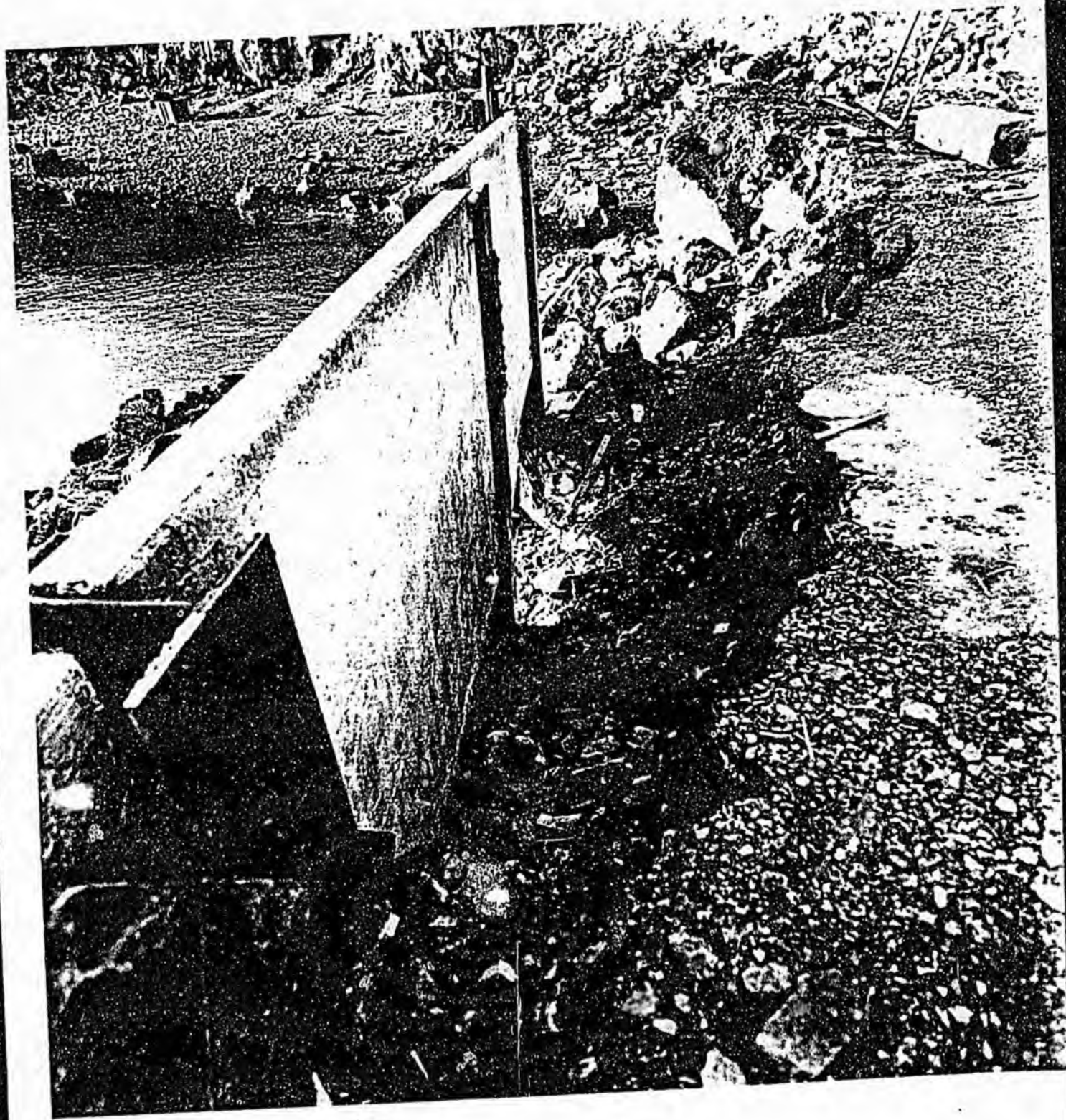
Kodisk, Alaska PIER 3 West wing wall on or about 1-28-80
