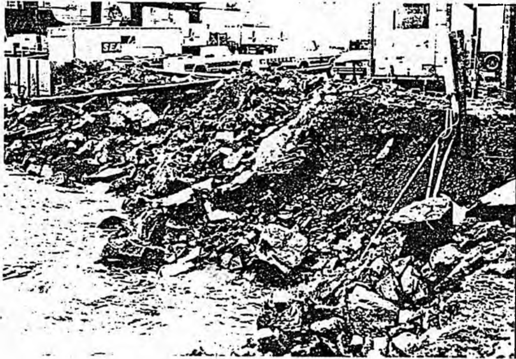
Photo No. 12: Slope erosion northerly of east wingwall. Note location of creosoted piling originally stored on top of bank.
