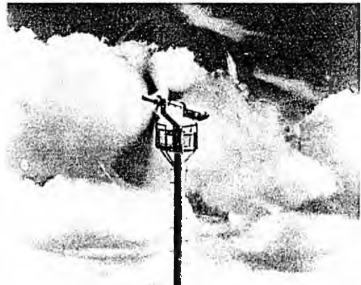
Windstream 25 in operation. Rotor is of the down wind type.
