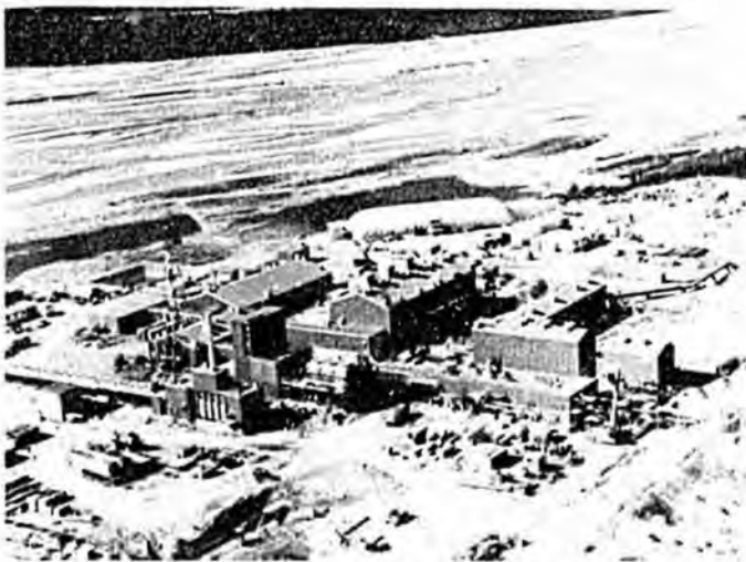
Pump Station 10 - Isabel Pass, Alaska Range
