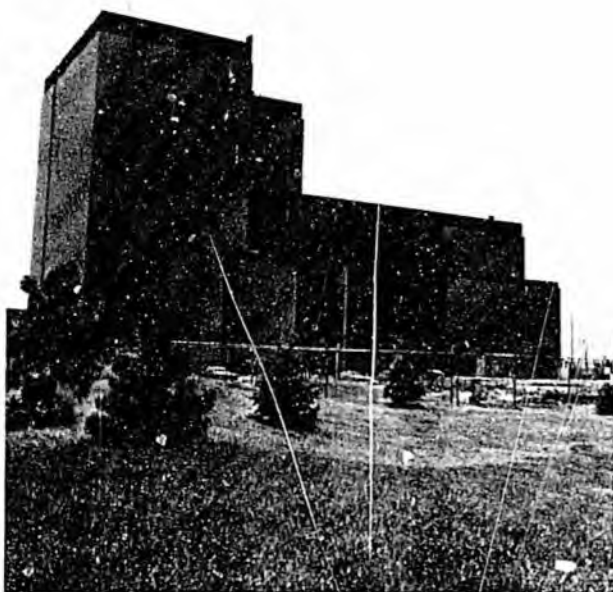
Fort St. Vrain Nuclear Generating Plant nearing completion near Platteville, Colorado.
