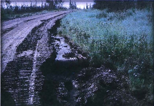
Failing Drainage
