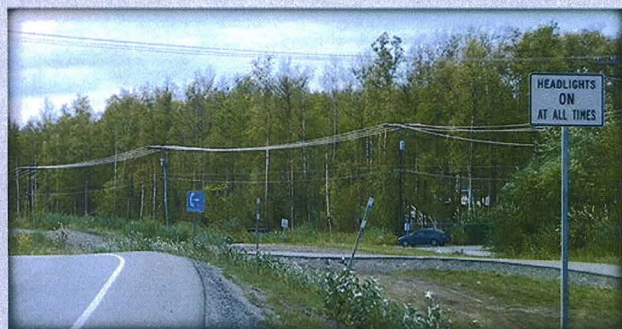
One of 47 signs installed in 2011 within four Safety Corridors. Photo by Brendan Dougherty, Alaska DOT&PF
