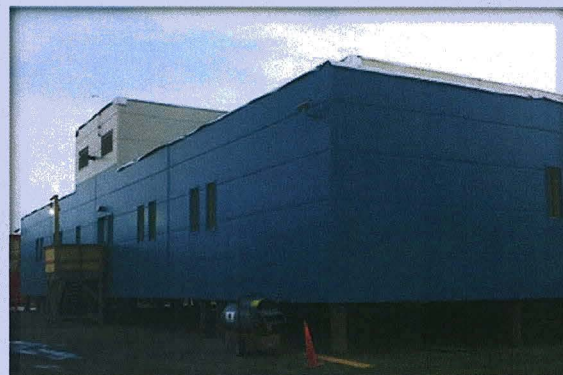
Bethel Youth Facility Photo by Alaska DOT&PF
