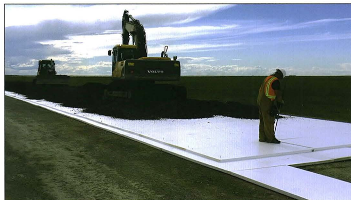
DALTON HIGHWAY/RECONSTRUCTION MP 401-414, BRICE INC.
