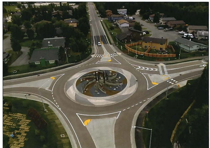
KLATT ROAD ROUNDABOUT, FINISHING EDGE CONCRETE, QAP
