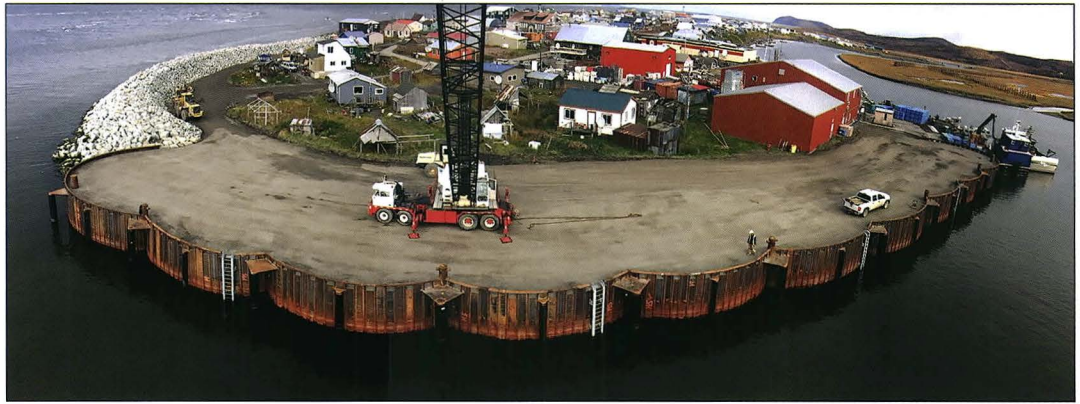
UNALAKLEET REVETMENT PHASE III, ORION MARINE GROUP
