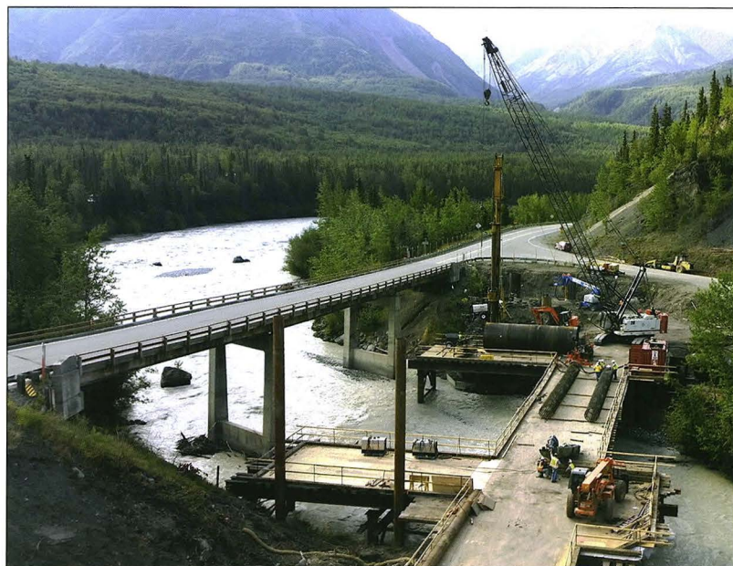
GLENN HIGHWAY CHICKALOON BRIDGE REPLACEMENT, HAMILTON CONSTRUCTION ALASKA CO.
