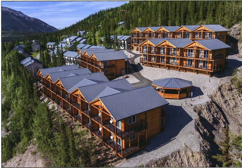
RIVERVIEW AT THE BLUFFS-DENALI, KLEBS MECHANICAL
