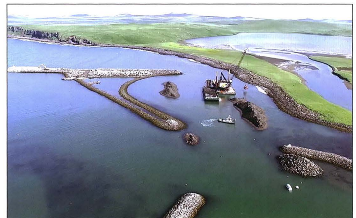
ST. PAUL BREAKWATER REPAIR AND MAINTENANCE DREDGING, KIEWIT INFRASTRUCTURE WEST CO.
