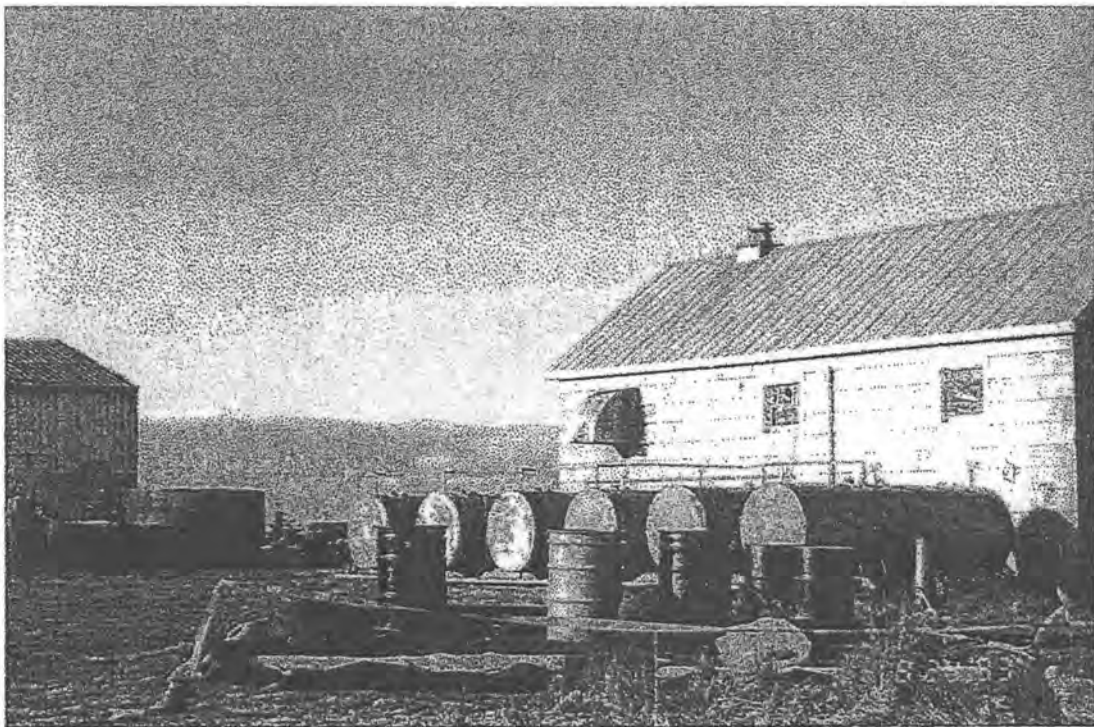
Figure 5. Tank Farm/Power Generation Building at Middleton Island
