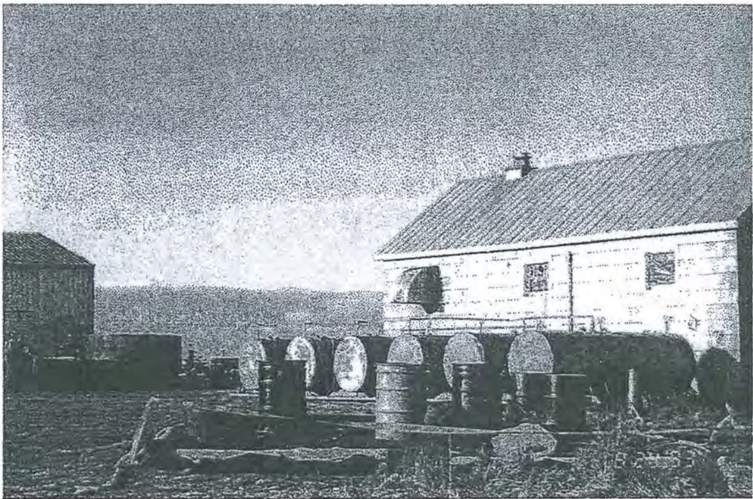
Figure 5. Tank Farm/Power Generation Building at Middleton Island
