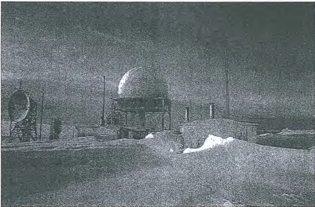
Figure 7. Typical Radome at a DEW Line Site in Winter
