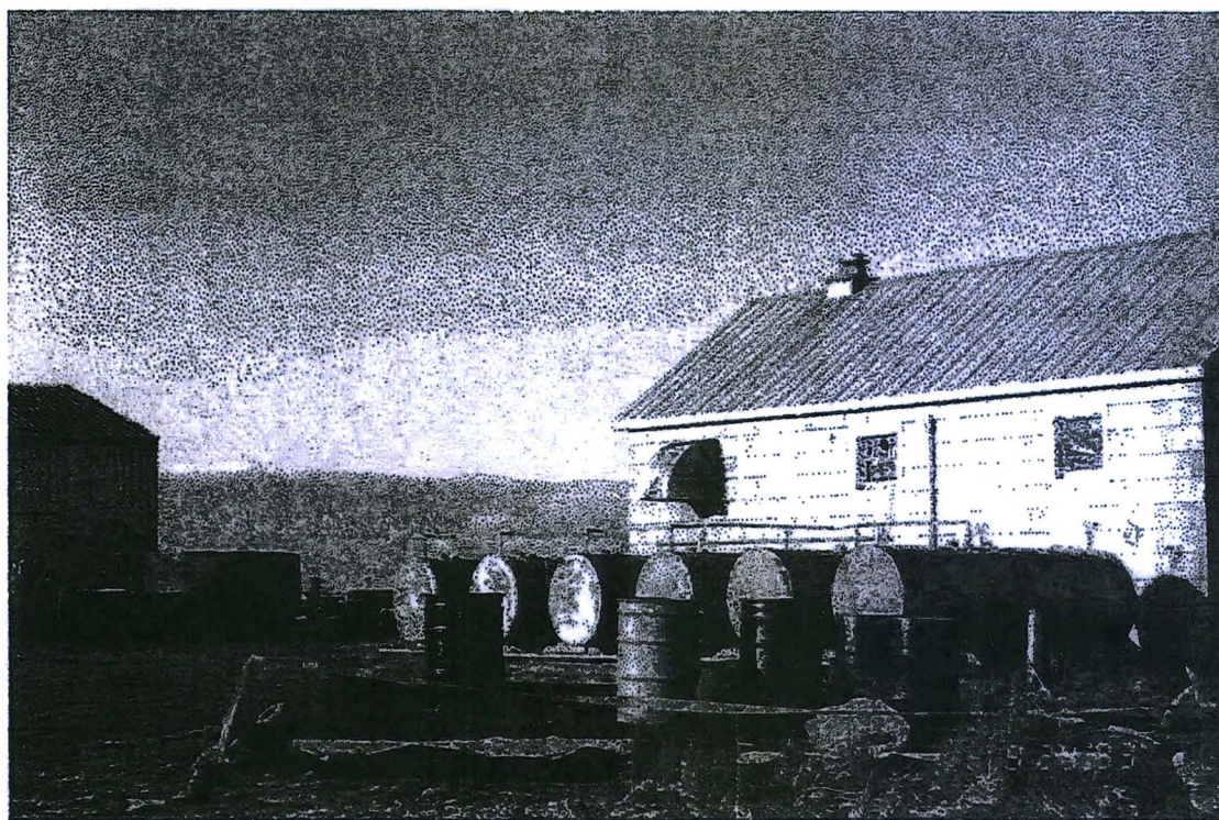
Figure 5. Tank Farm/Power Generation Building at Middleton Island
