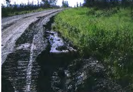
Failing Drainage
