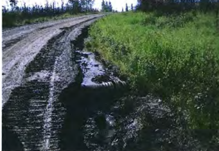
Failing Drainage
