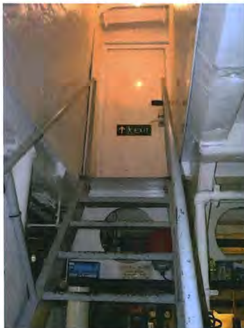
Photo 8-1 : Staircase from MSD Room (Hold Deck) To Second Deck Crew Quarters
