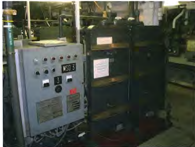
Photo 7-1 : Skid Mounted Single Pass 12MX bookcells and Control panel
