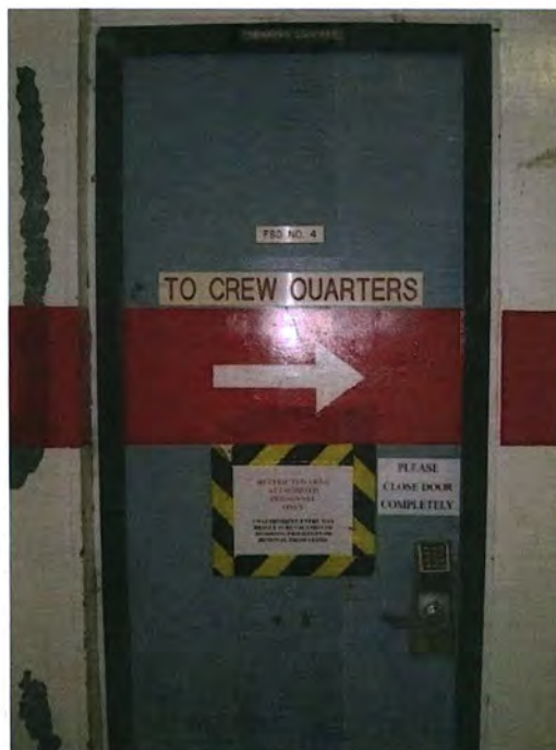
Photo 8-3 : Fire Safety Door #4 leading to open Main Deck (Viewed from Vehicle Deck)
