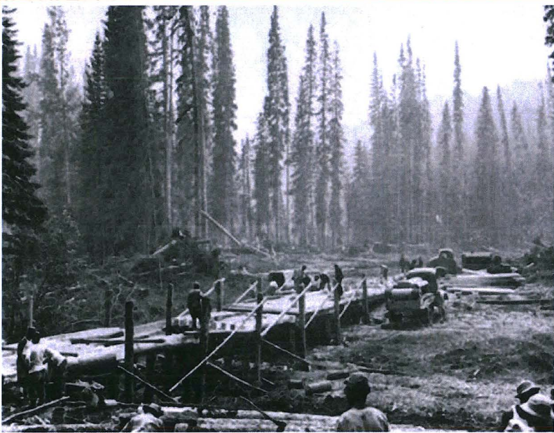
Black engineers build a trestle bridge during the construction of the Alaska Canada Military Highway. Black G.I.s made up roughly forty percent of the estimated 11,500 Army troops who in just nine months completed a wilderness highway linking Alaska with the contiguous United States.
