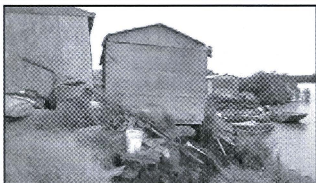
Figure 22.8: One effect of the reduction in Alaska sea ice is that storm surges that used to be buffered by the ice are now causing more shoreline damage. Photos show infrastructure damage from coastal erosion in Tuntutuliak (left) and Shishmaref, Alaska (right). (Photo credits: (left) Alaska Department of Environmental Conservation; (right) Ned Rozell).
