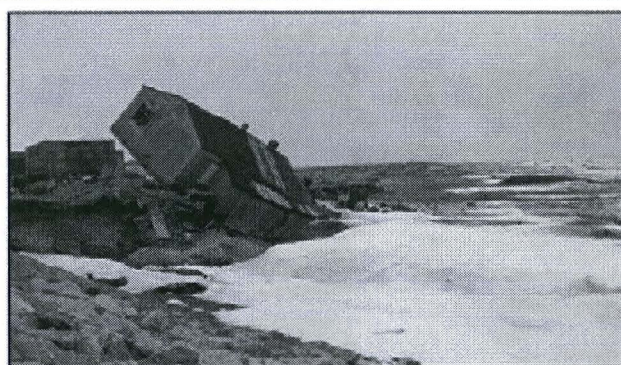
Figure 22.8: One effect of the reduction in Alaska sea ice is that storm surges that used to be buffered by the ice are now causing more shoreline damage. Photos show infrastructure damage from coastal erosion in Tuntutuliak (left) and Shishmaref, Alaska (right). (Photo credits: (left) Alaska Department of Environmental Conservation; (right) Ned Rozell).
