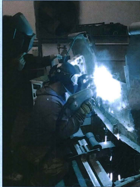
At right, weekend welding instruction in Point Lay
