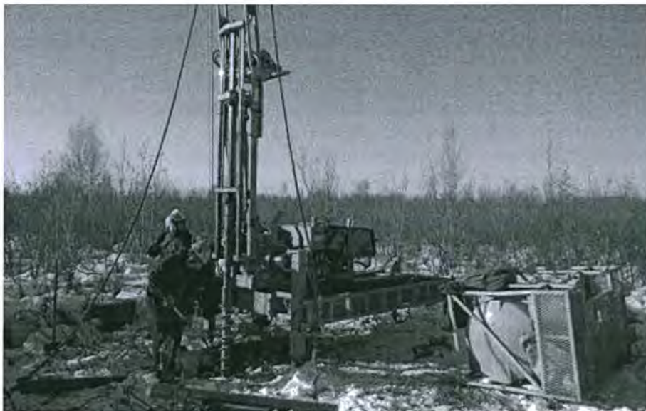
Photo 1: Borehole drilling with a heli-drill rig
