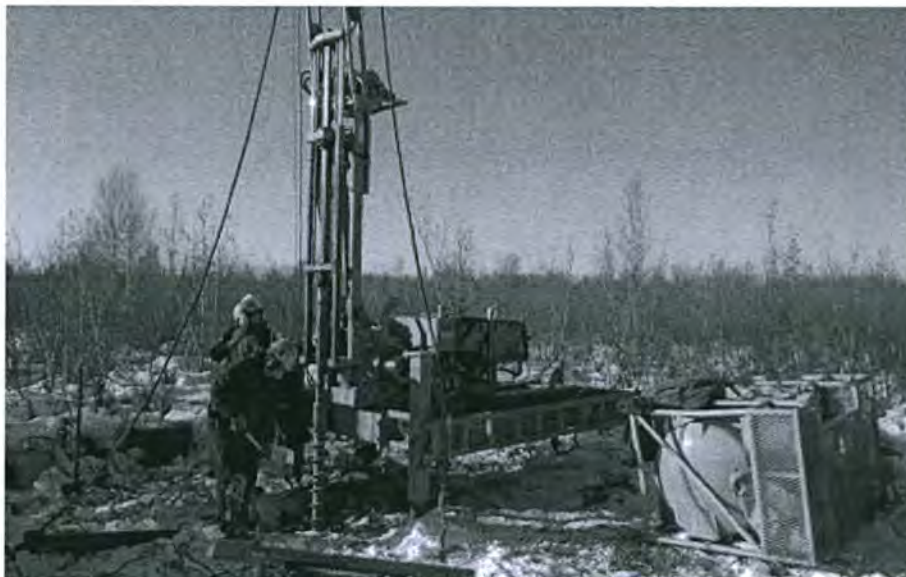
Photo 1: Borehole drilling with a heli-drill rig
