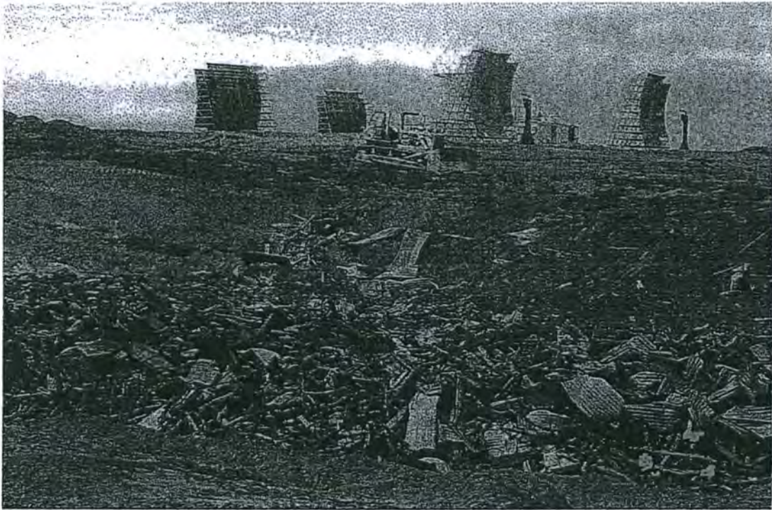
Figure 6. DEW Line Site at Port Heiden (ANCSA selected, not conveyed)
