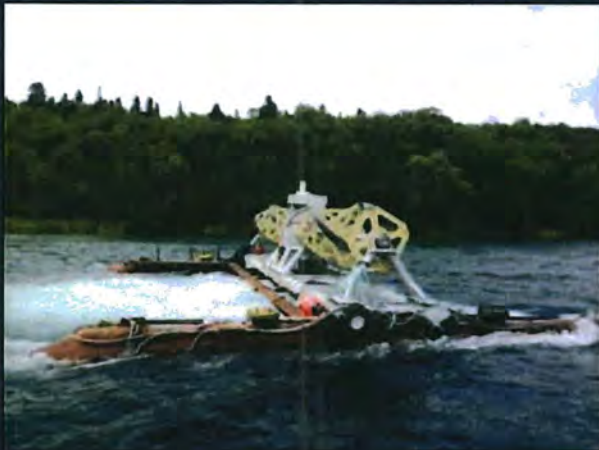
ORPC Turbine in the Kvichak River
