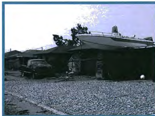
Boat rests on roof of Louisiana home after Hurricane Katrina, August 2005
