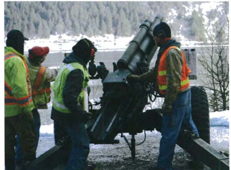
Southcoast Maintenance Shooting down avalanches on Thane Road.
