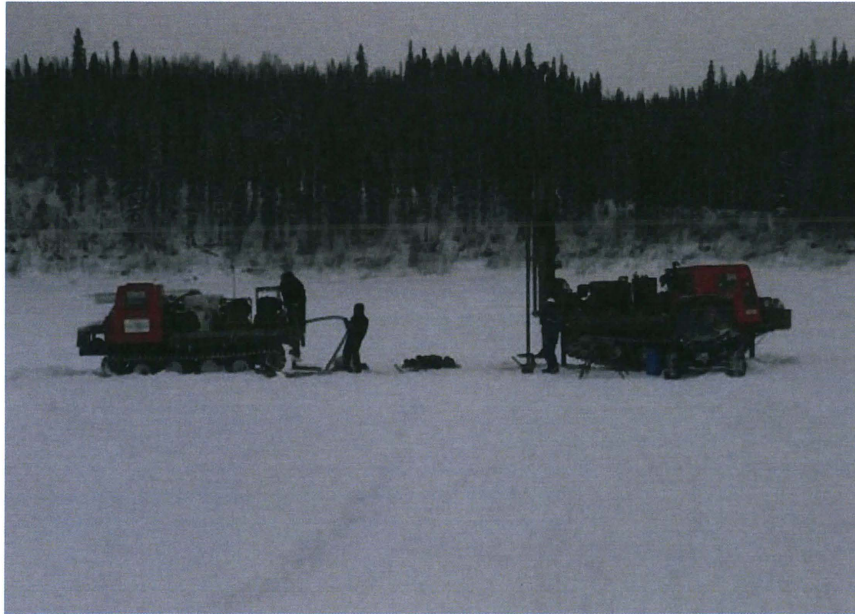
Photo 1: A track mounted drill rig and support vehicle on ice (Approximate weight: 35,000 lbs).
