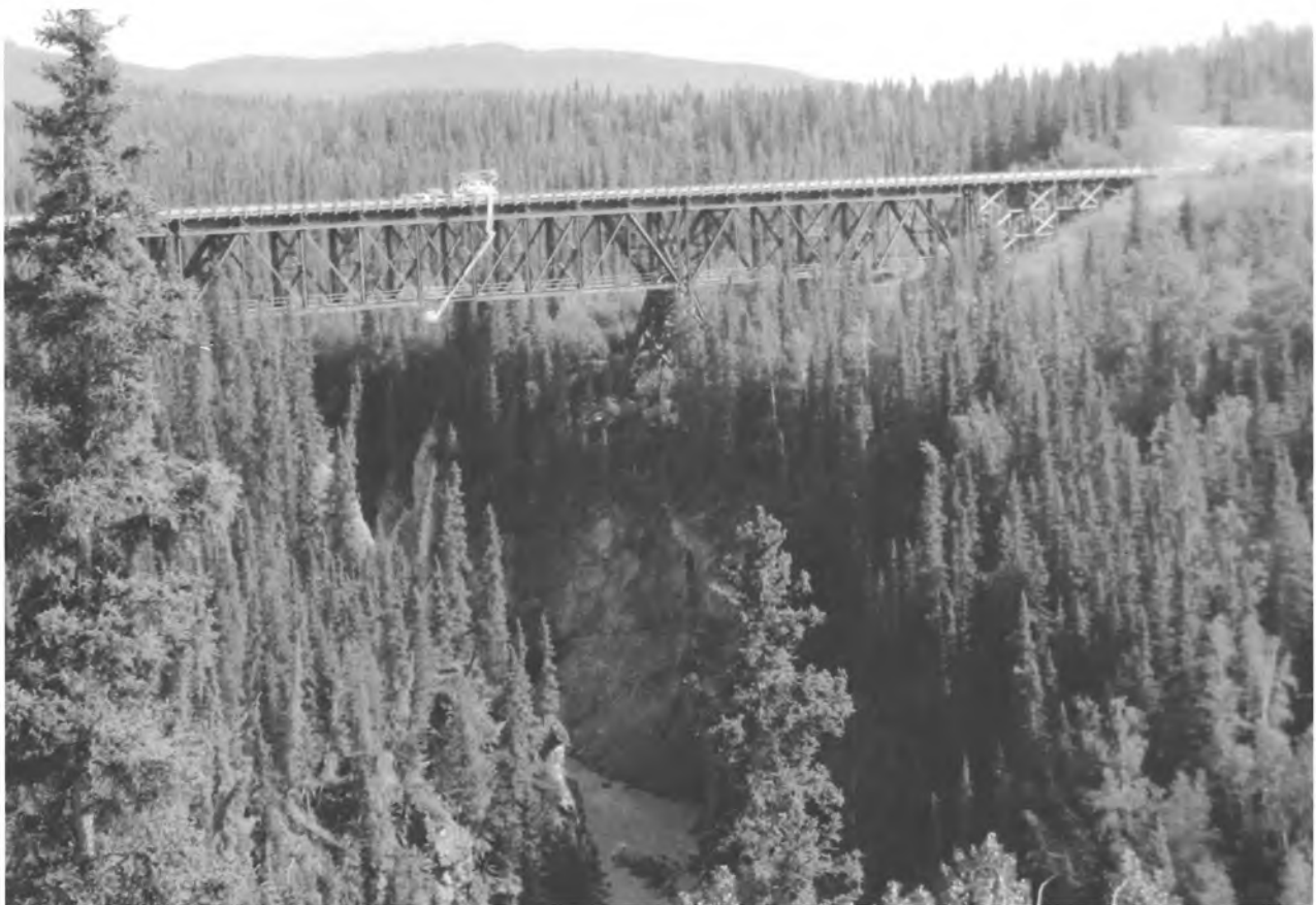
Figure 11. DOT Inspectors on the Kuskalana Bridge
