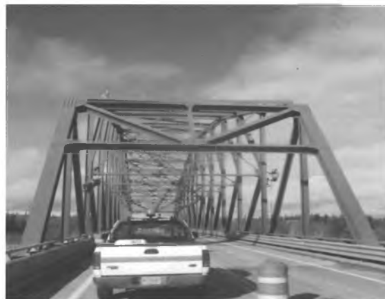
Figure 7. Consulting Engineers Inspect the Rex Bridge
