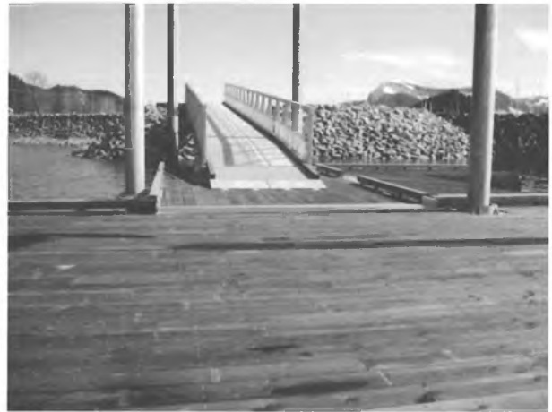
Figure 20. Hoonah Seaplane Float Ramp
