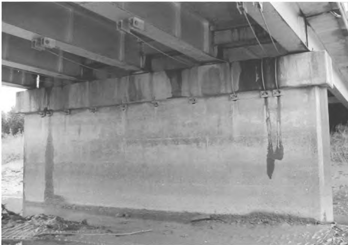
Figure 10. Phase 1 Seismic Retrofit Using Cable Restrainers Twenty Mile River Bridge
