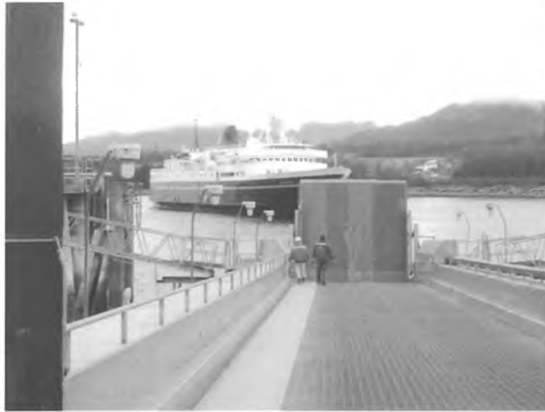
Figure 19. Ketchikan Ferry Terminal Ramp
