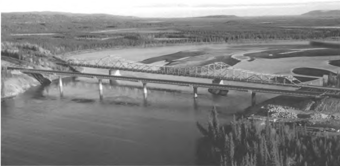
Figure 16. New and Old Tanana River Bridges
