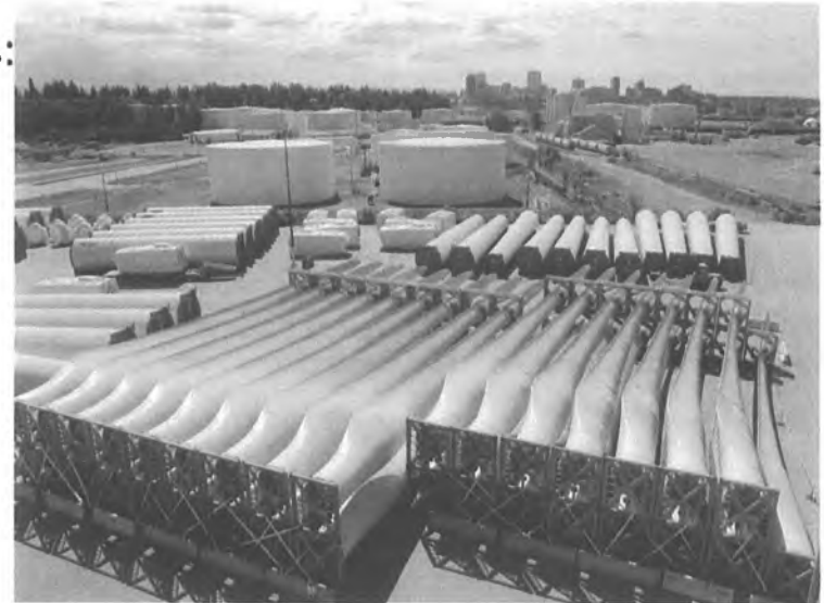
Fire Island Wind Turbines (Dry Barge Berth Used to Transport)
