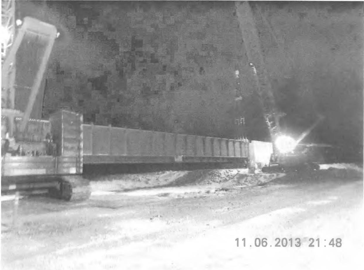
Last bridge girder erected
