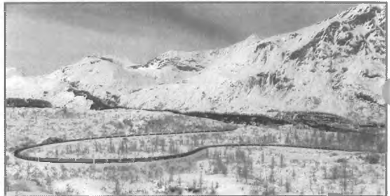
ARRC export coal train climbing to Grandview. This area requires significant communications systems to support PTC.
