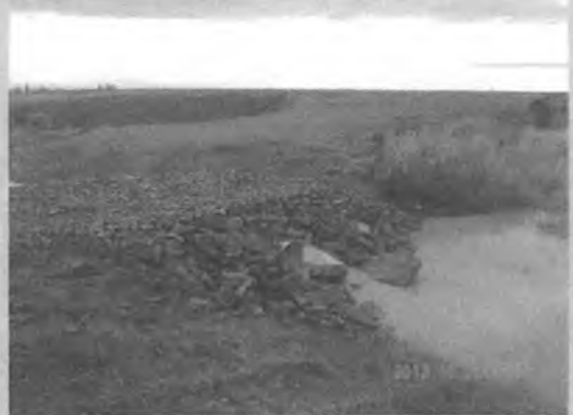
Drainage repair and improvements at BMBF pad
