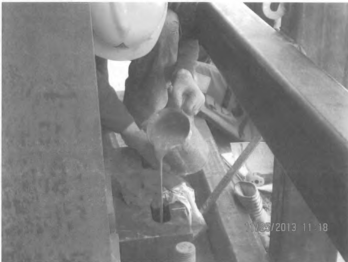
Setting anchor bolts
