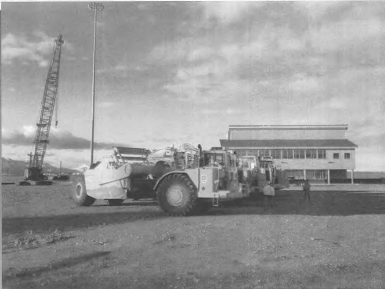
Barge dock staging area
