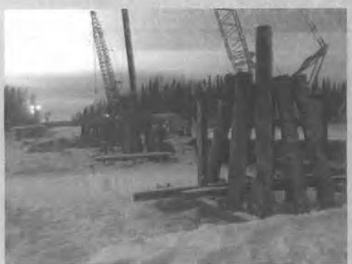
Driving Pile on Diamond Lake Outfall Bridge
