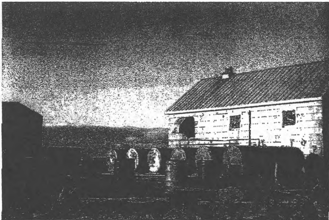
Figure 5. Tank Farm/Power Generation Building at Middleton Island
