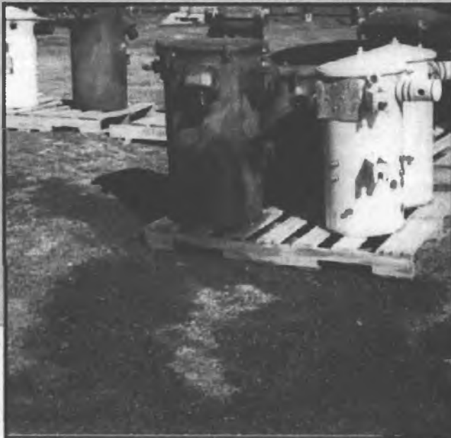
Transformers containing PCBs can release hazardous chemicals into soils.
