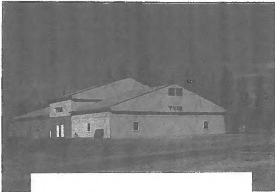
New TVSA Classroom/Range (shell built in 2008-09)
