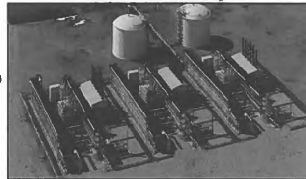
SCLNG Plant and Storage
