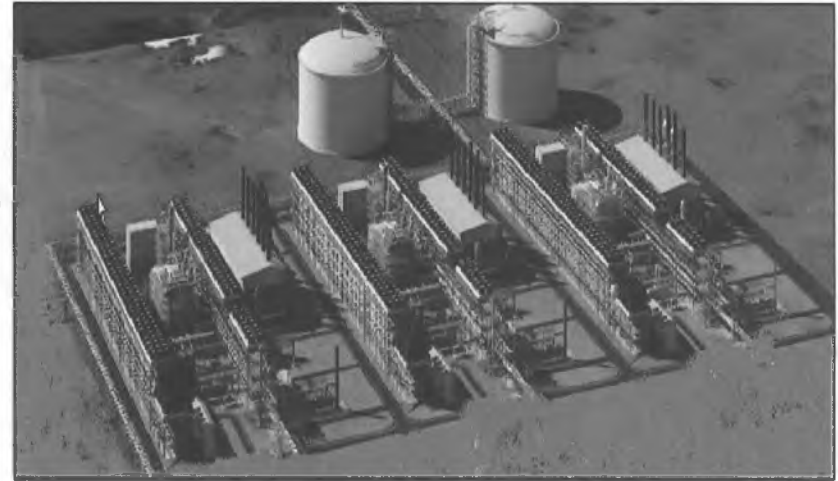
SCLNG Plant and Storage
