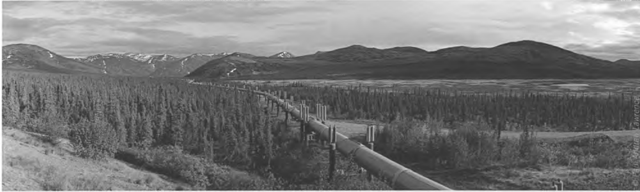
Trans Alaska Oil Pipeline through the Brooks Range of Alaska
