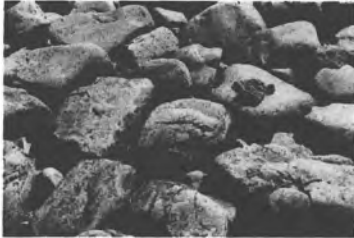
A well-integrated boulder armor near the Cape Douglas site. The stocking hat measures 22 cm across.
