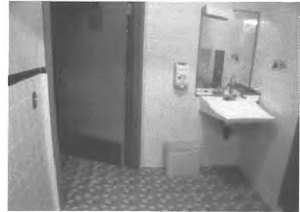
Ketchikan Pioneer Home Third Floor Remodel Bath Before
