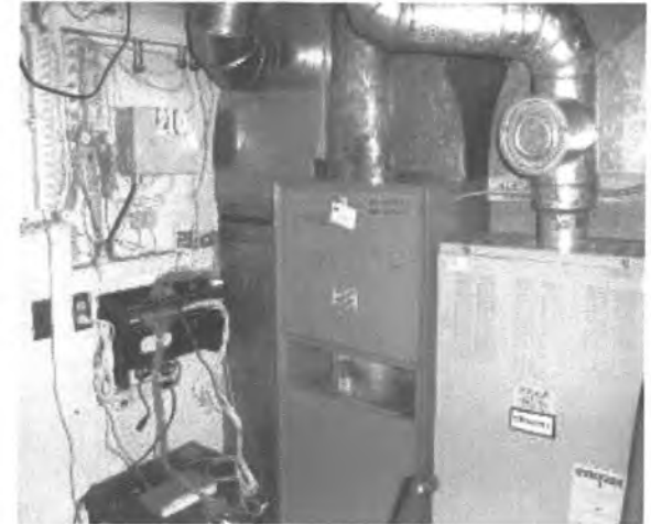
Sitka Public Health Furnace Replacement Before
