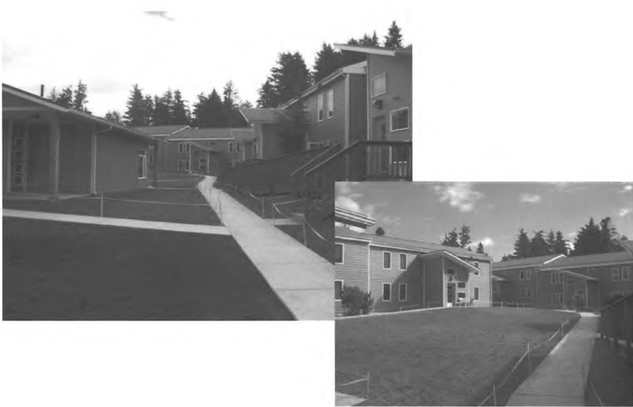
Fir Terrace Renovation Project – Kodiak – Vitus Development Group - Rehabilitation of 62 Units - 2009
