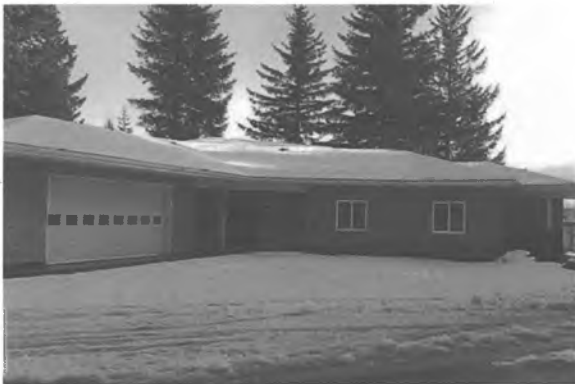
Special Needs Housing Grant funded project from FY2009 Cycle
