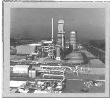
GTP & Transmission Lines
