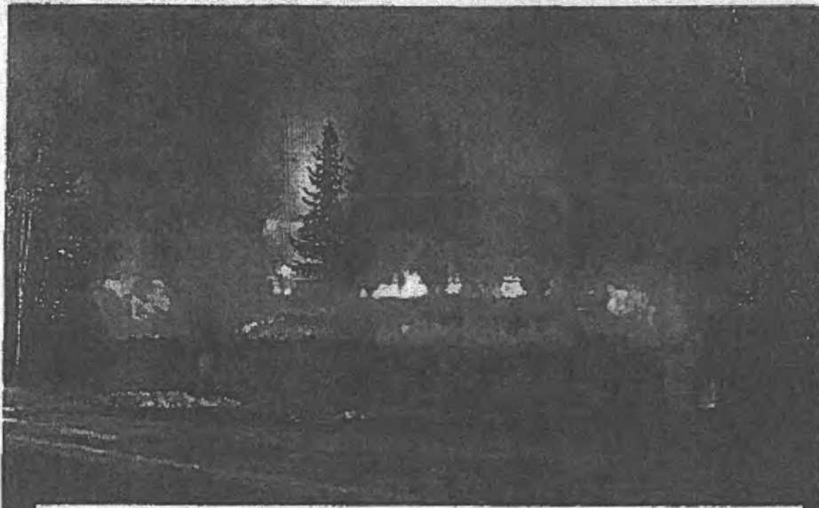
TVSA Clubhouse/Range, built in the 1930's, destroyed by fire on 3/31/2007
