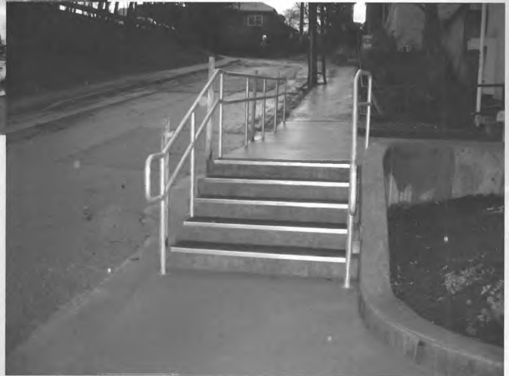
Juneau Alaska Office Bldg Sidewalk After
