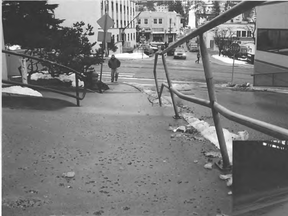
Juneau Alaska Office Bldg Sidewalk Before
