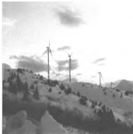
Pillar Mountain Wind Phase 1 & 2, and Battery Photo Courtesy of Kodiak Electric Association
