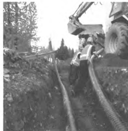
Heat Recovery System installation - Hoonah Alaska Energy Authority
