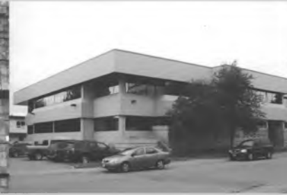
The Trust purchased a 29,000-square-foot Class A building in Anchorage that provides lease income and office space for the TLO.
