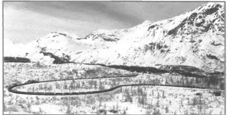
ARRC export coal train climbing to Grandview. This area requires significant communications systems to support PTC.
