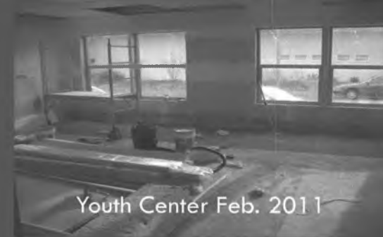
West Side of Building Feb. 2011
