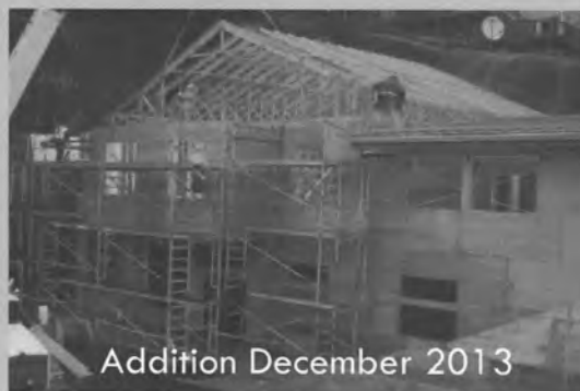
Addition Second Floor December 2013
