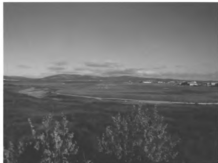
Nome Airport - new runway safety area constructed on Runway 3. DOT&PF Project Photo
