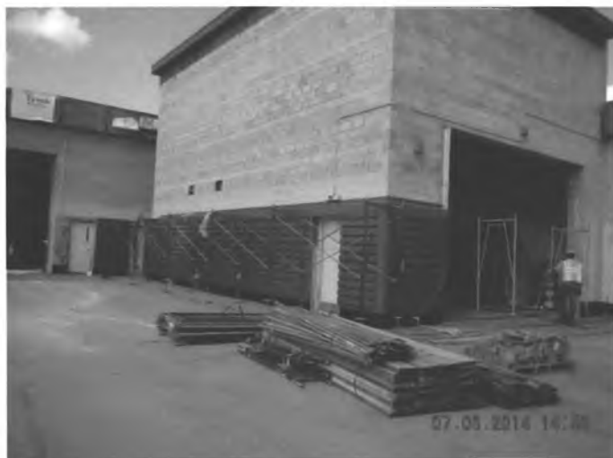
ARFF building at FAI was rehabilitated in 2014
