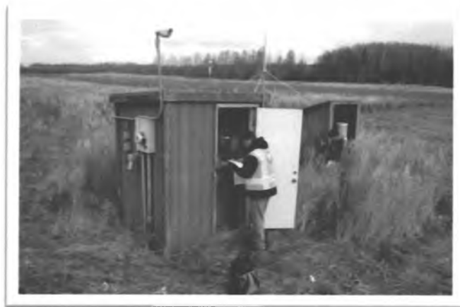
Airport inspection in Holy Cross this past summer. Photo credit - Jason Sakalaskas, DOT&PF
